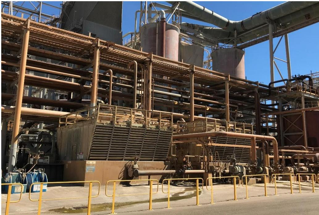
**Figure 19: Calcination cooling towers**
