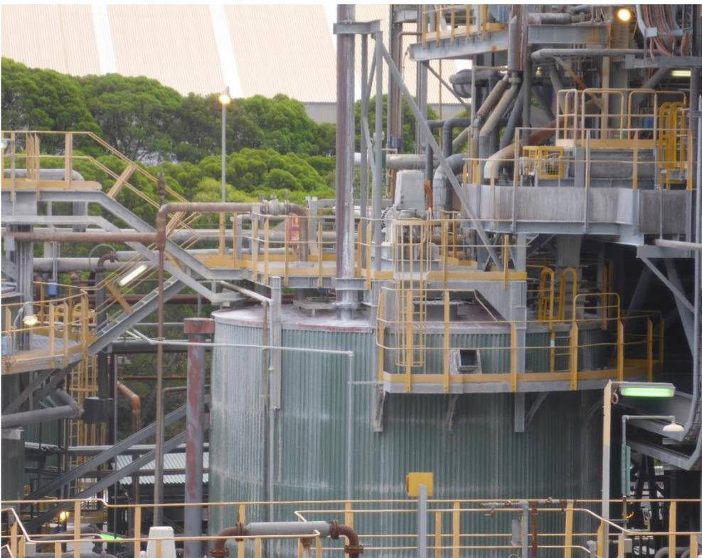
Figure 13: Liquor Burning Slurry Mixing Tank (48A)
