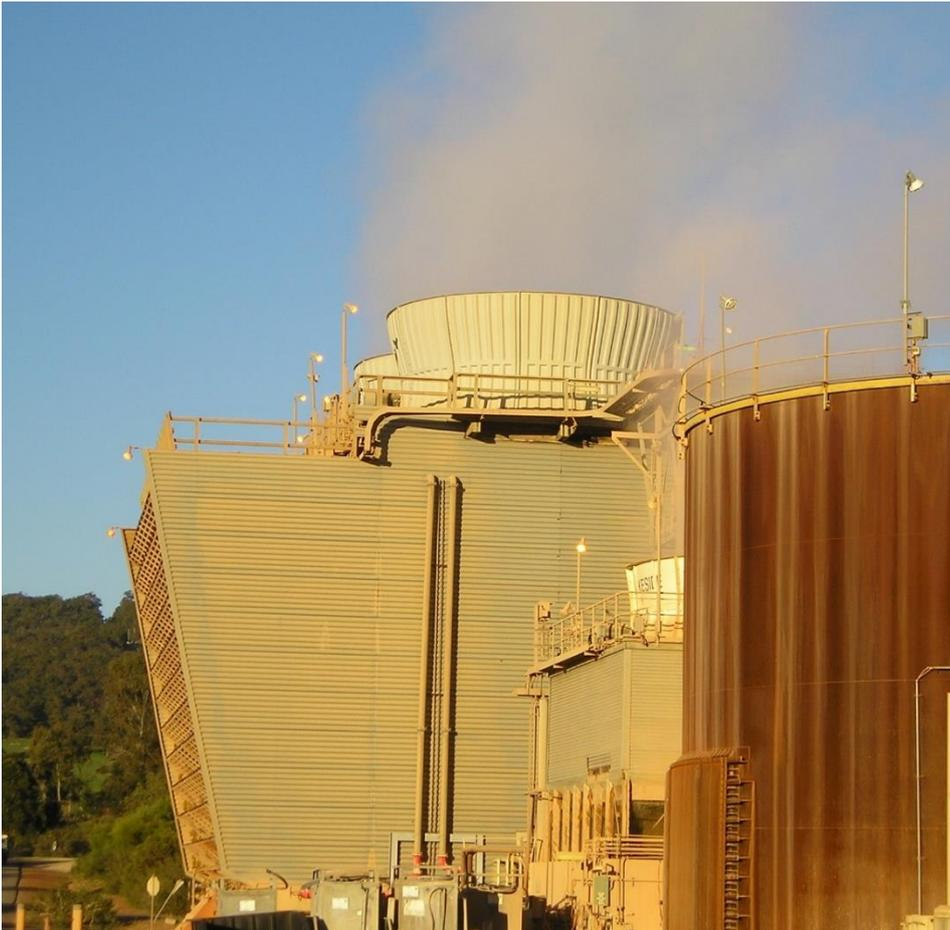
**Figure 9: Precipitation Cooling Towers**
