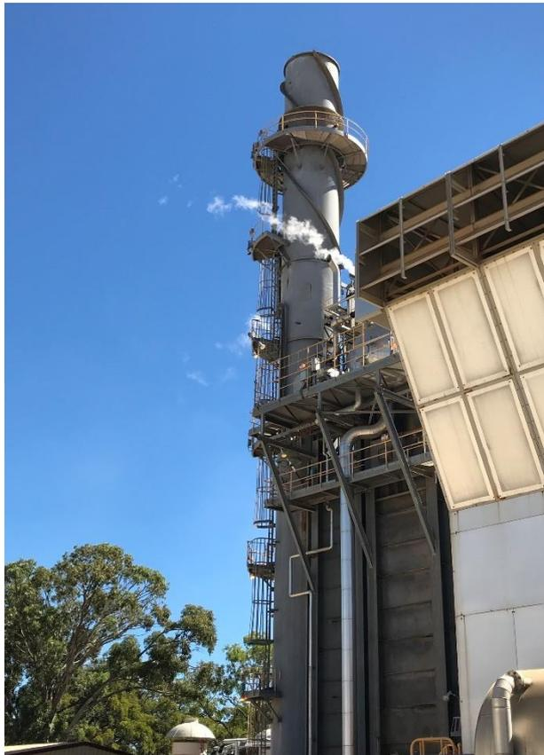
Figure 21: GT/HRSG stack
