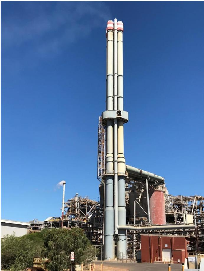
**Figure 16: Calcination multi-flue stack (includes Calciner 1-3 LVV)**
