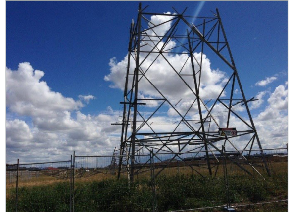
Transmission Line Tower T064 removal.
