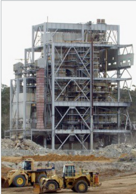
The remaining power station structure.
